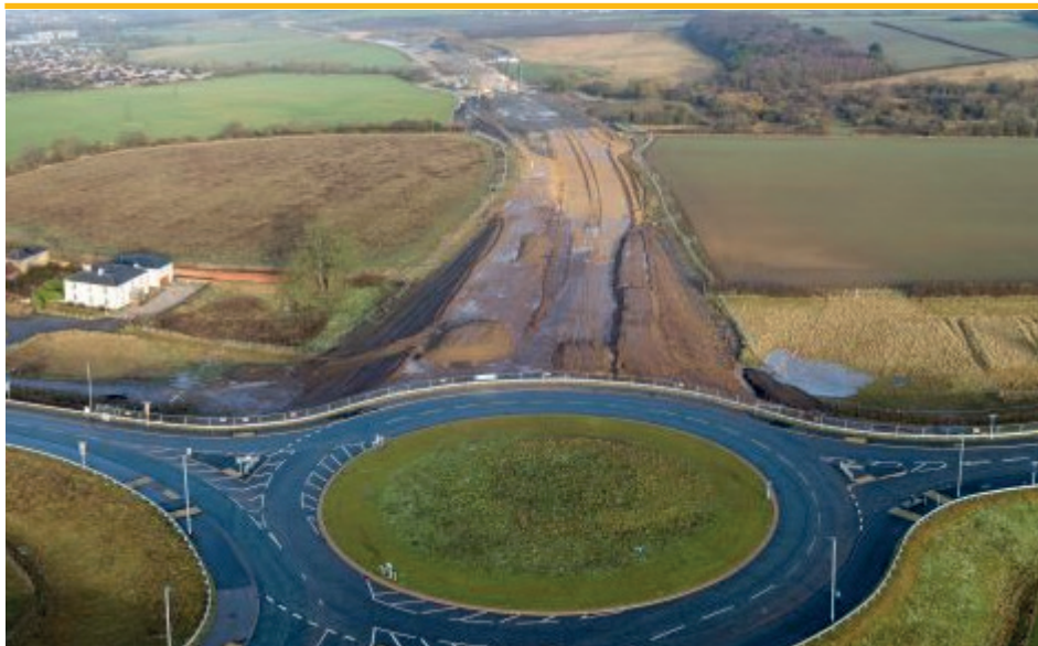
ELOR Drone View of Manston Lane Tie-in Junction 6 – Mar 2021
