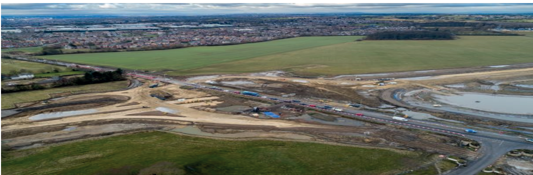
ELOR Drone View of York Road A64 Roundabout Mar- 2021
