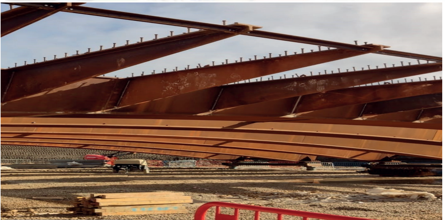
Country Park Underpass Mar 2021
