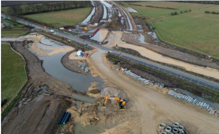
ELOR Drone View of The New Skeltons Lane Roundabout Junction 3 - Mar 2021
