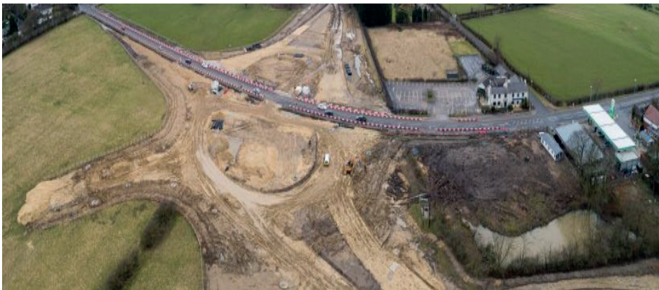
ELOR Drone View of Junction 2 The New A58 Roundabout Site – Mar- 2021
