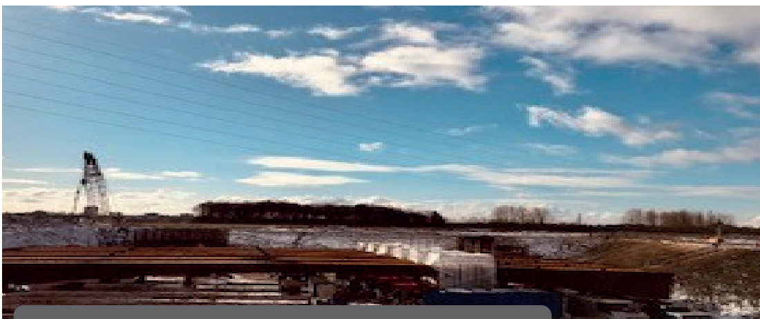
Country Park Underpass - Mar 2021
