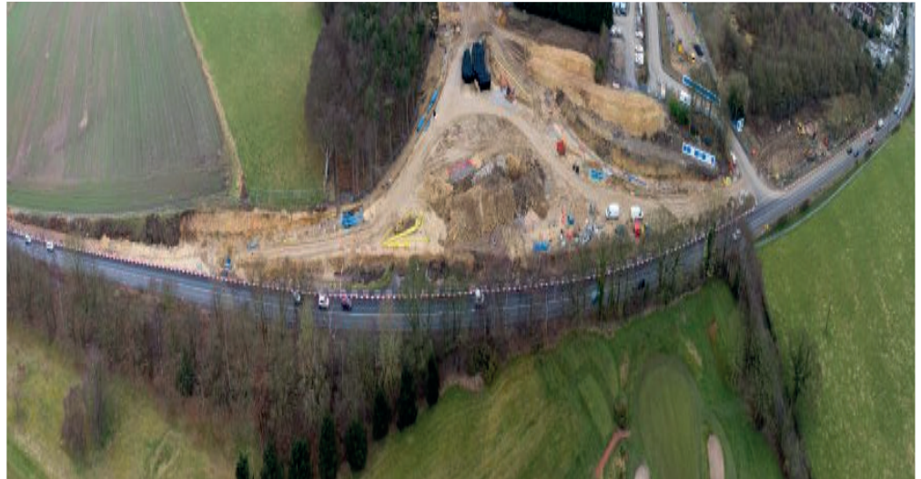
ELOR Drone View of Junction 1 The New A6120 Roundabout Site – Mar 2021
